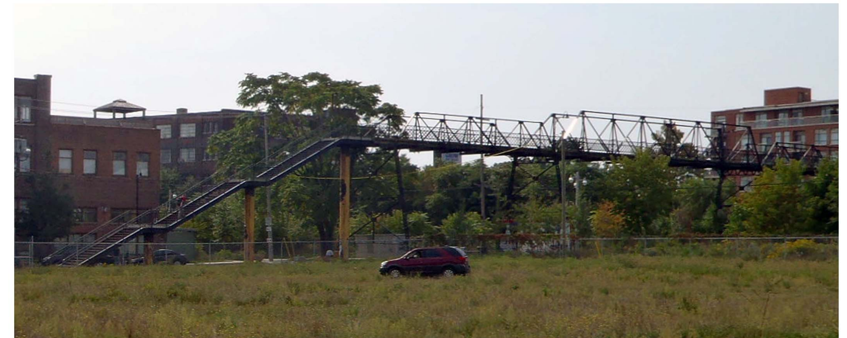
Existing Pedestrian Bridge
